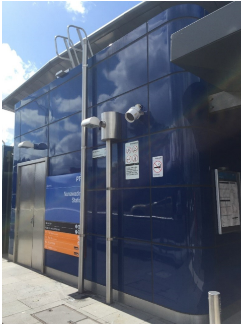
Figure 8: Nunawading Station – Prefabricated buildings provide ease of installation and improved quality control of workmanship. Vitreous enamel cladding provides a hardwearing and attractive finish
