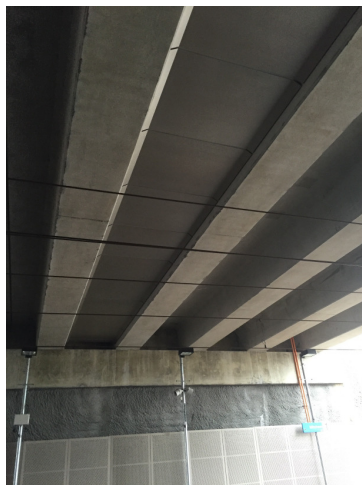
Figure 7: Mitcham Station – Services were concealed behind cladding (second gap) to avoid unsightliness.
