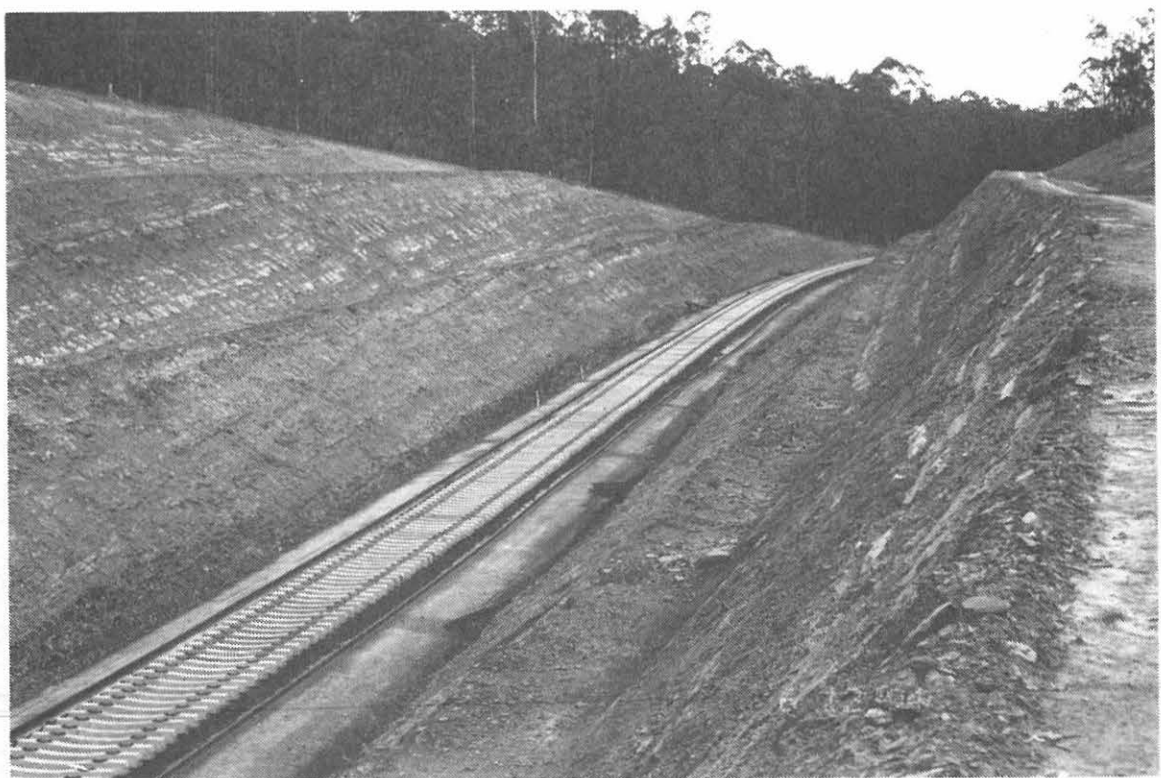
Fig. 4. Rappville Deviation. Deep cutting to flatten grade and remove sharp curves.
