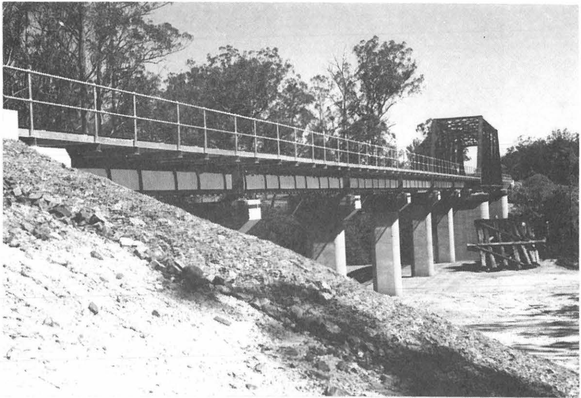
Fig. 3. Kungala. Sherwood Creek. Timber transom top approach spans replaced by concrete & steel structure.
