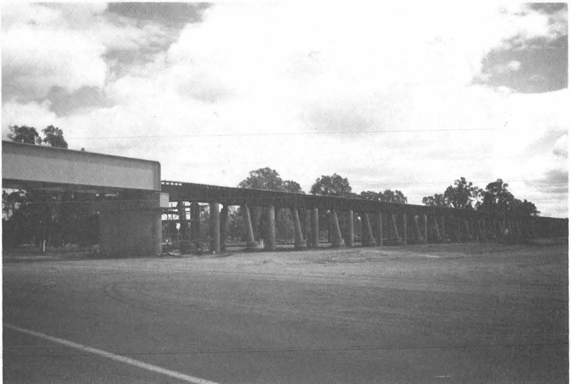
Fig. 8. Wagga Wagga Viaduct. After - Oura Rd - new steel span. Old steel trestles concrete encased with new intermediate concrete trestles.
