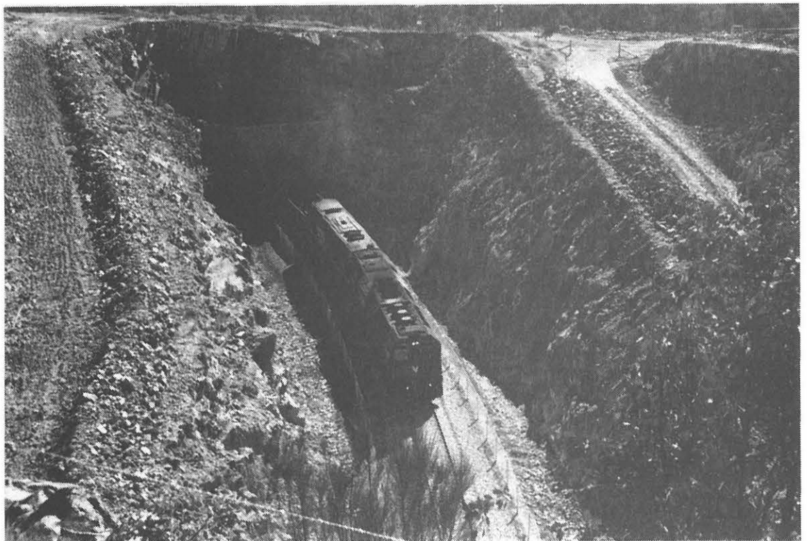
Fig. 10 Bethungra. First train through widened granite cutting between tunnels
