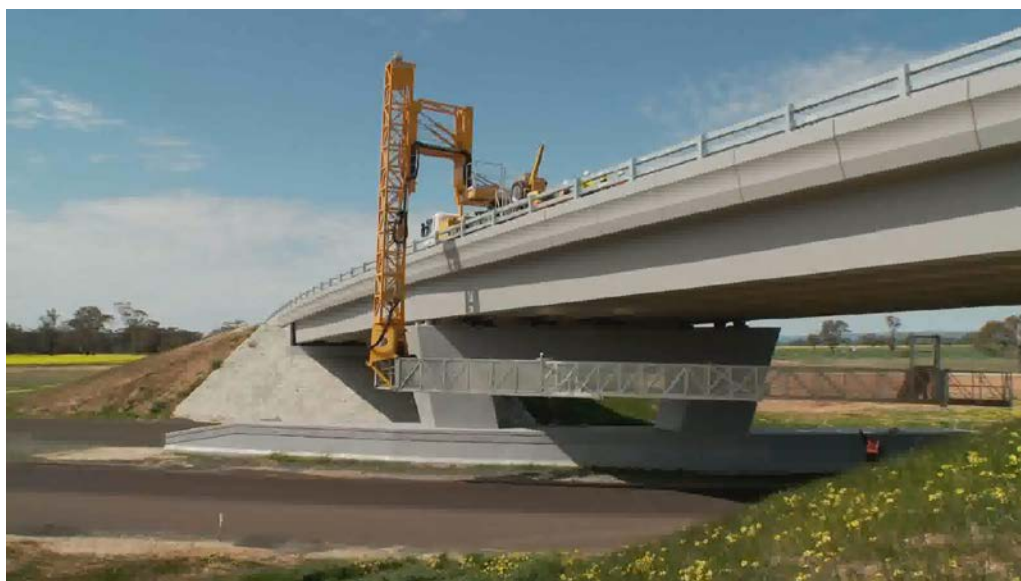
Figure 5 MBIP deployed under bridge on Nagambie Bypass
