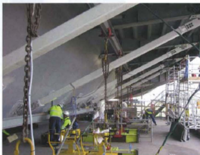
Figure 4 – Sloping props being installed to support steel bridge cantilever
