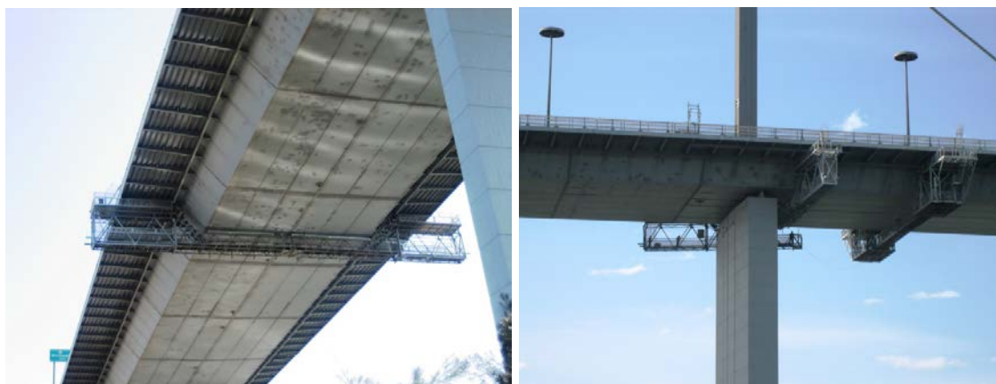
Figure 3 – Gantries suspended from steel bridge prior to recent strengthening project
