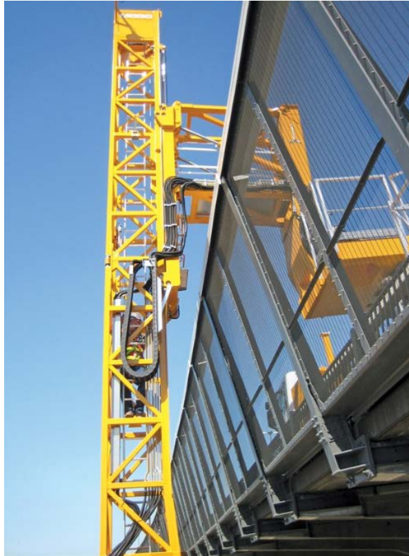
Figure 8 MBIP tower adjacent to 4m high Public Safety Barrier
