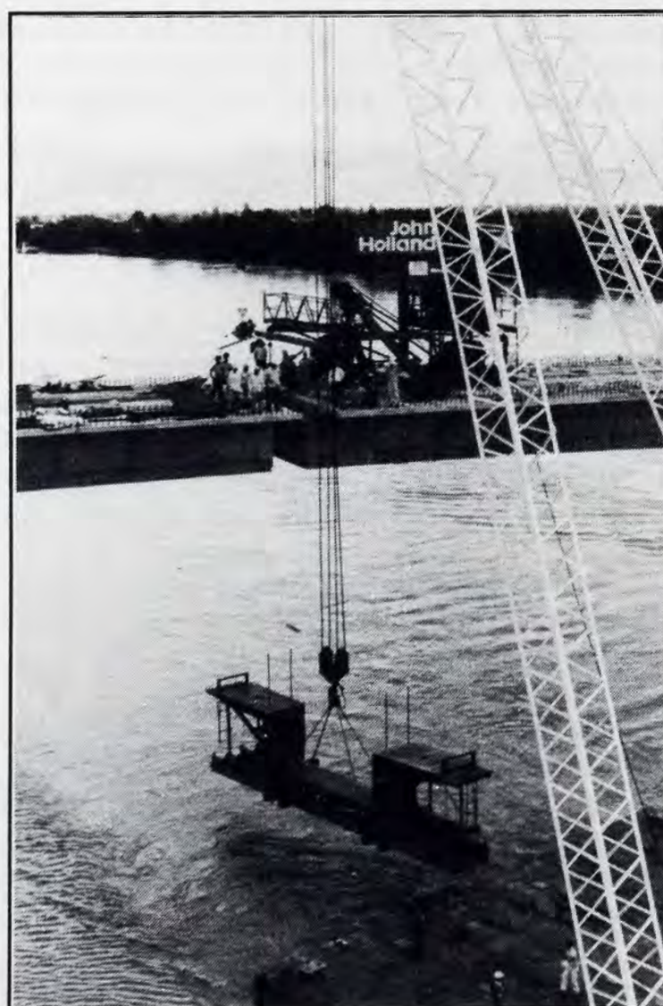
Putting the last segment in place
