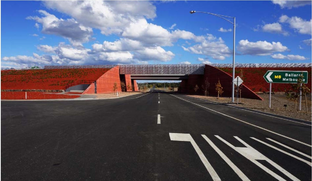
Picture 5: Western Highway at completion between Ballarat and Burrumbeet - Ballarat Avenue of Honour Remembrance Drive. 2015
