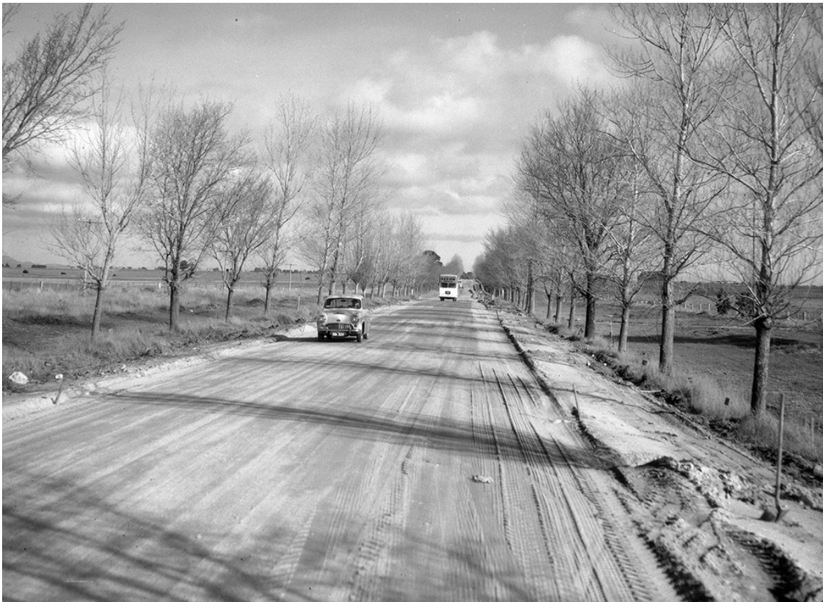
Picture 1: Western Highway under re-construction between Ballarat and Lake Burrumbeet. 1963
