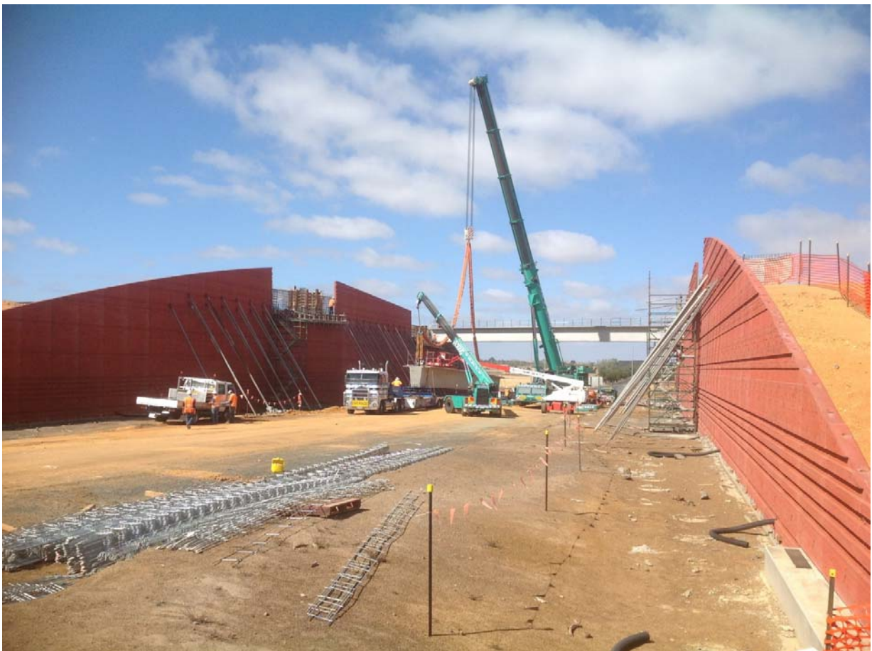
Picture 4: Western Highway under construction between Ballarat and Burrumbeet - Ballarat Avenue of Honour Remembrance Drive. 2014
