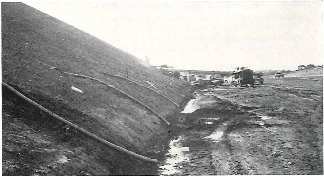
Plate 11—Drilling horizontal sub-surface drains at Mulgrave Freeway.
