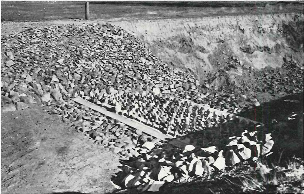
Plate 8—Completed drop structure near the co-axial cable.
