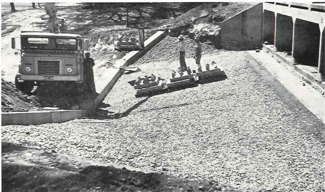
Plate 5—Filter layer spread level with top of upstream cap. The design of the precast concrete dissipator blocks to facilitate interlocking may be seen.
