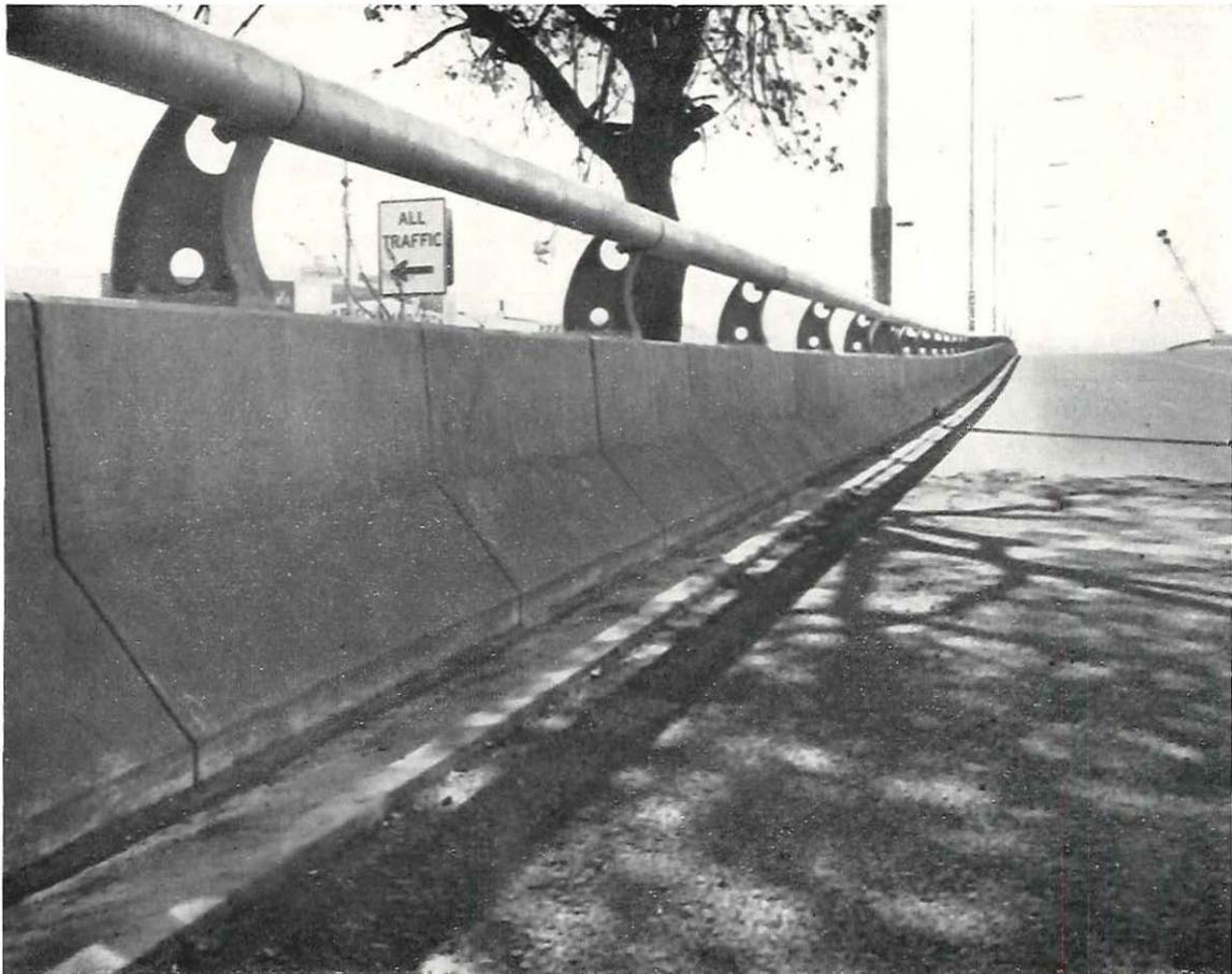
Plate 1—Precast concrete traffic barrier, West Footscray Bridge, Princes Highway West.
