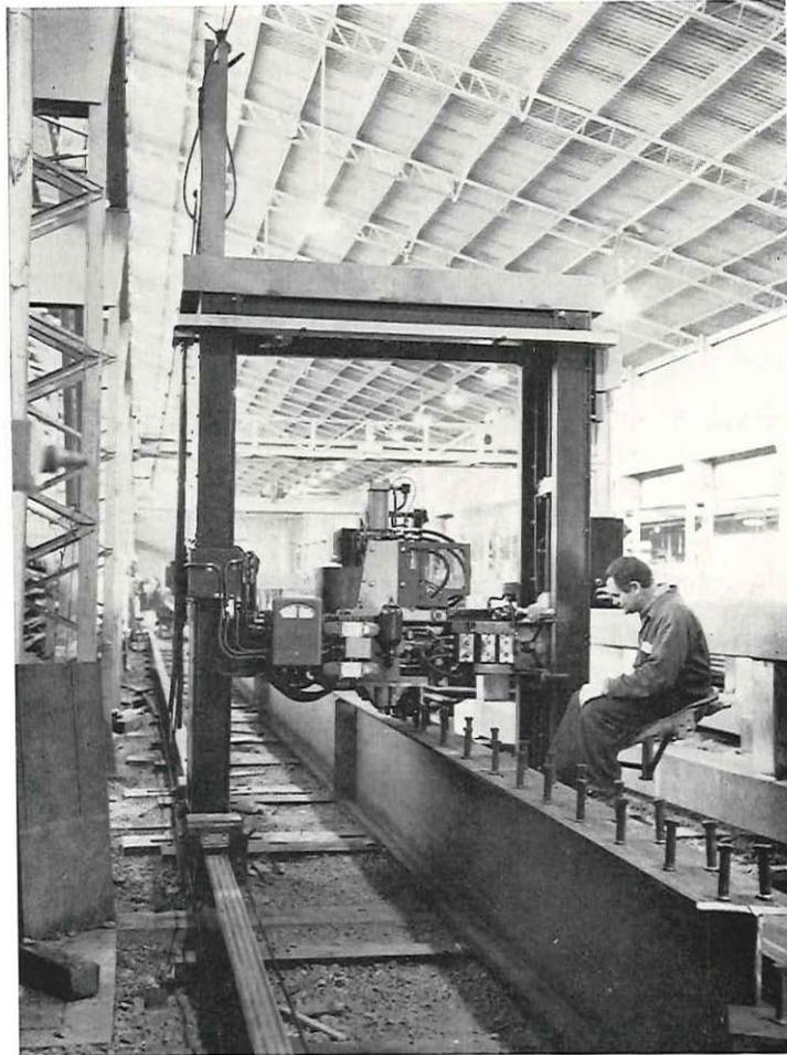
Plate 9—Production friction welding machine
