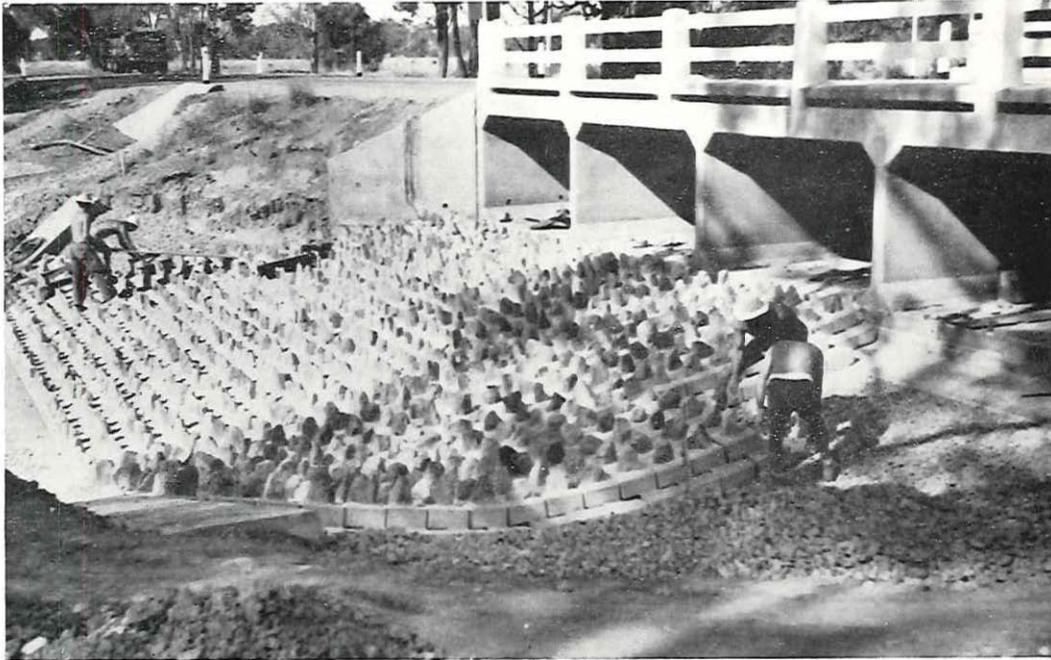
*Plate 6—Placing the dissipator blocks.*
